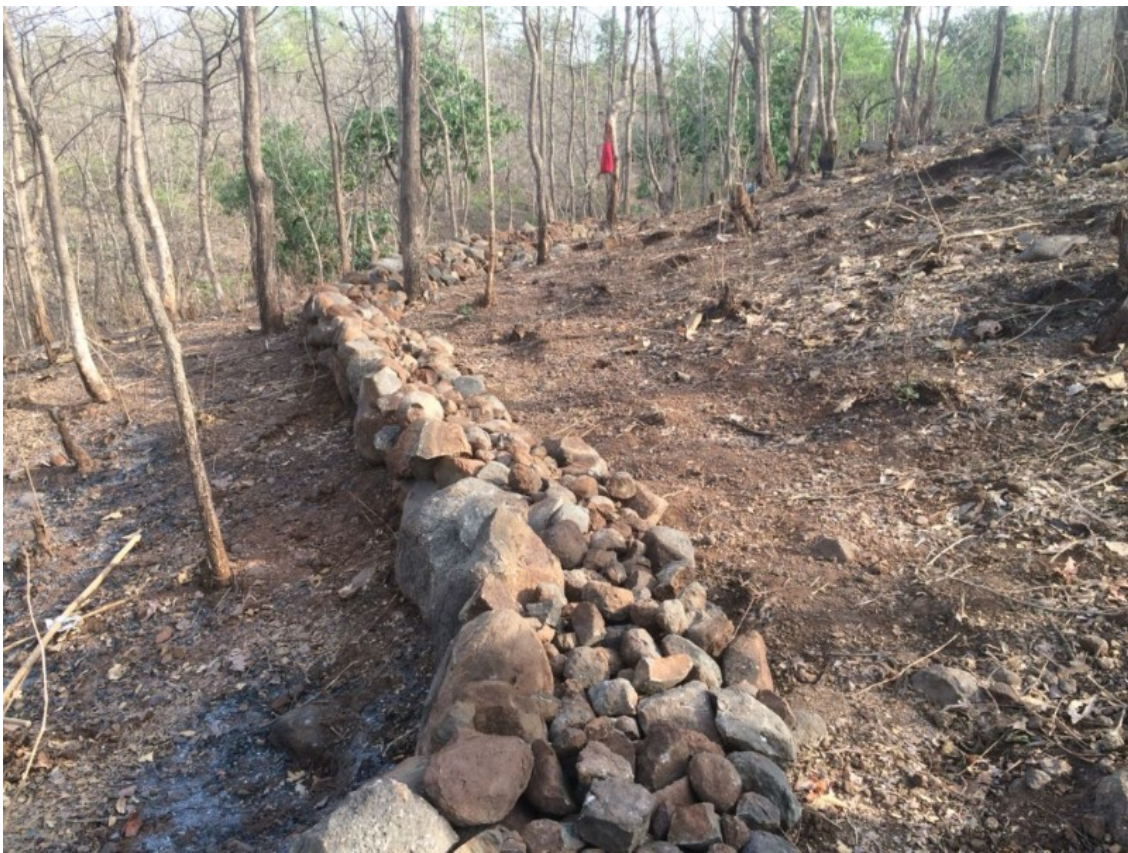
Results from the training - a rock swale to catch water and stop erosion
